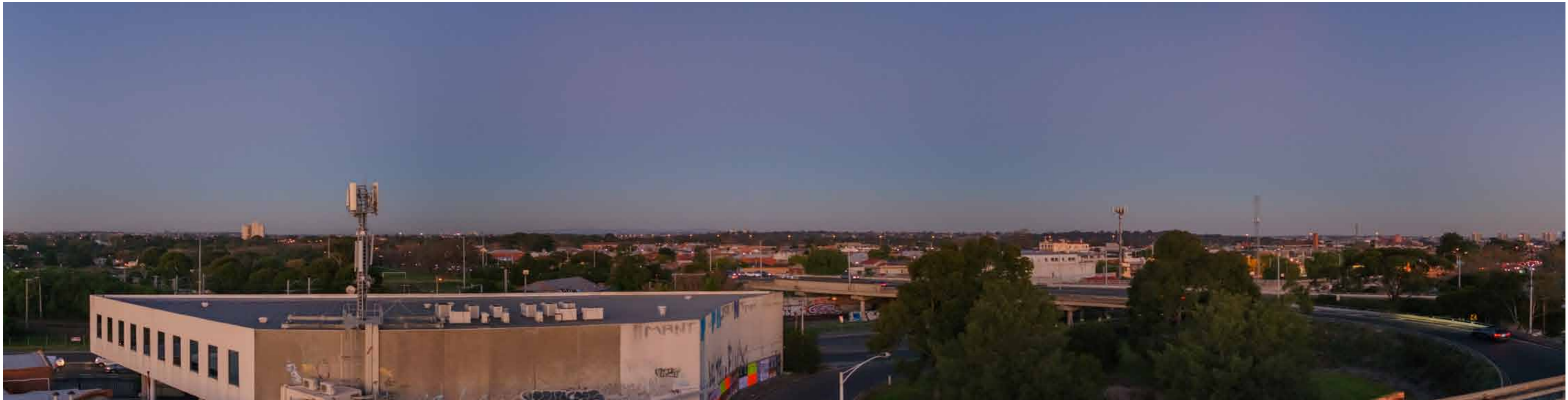
Level 5 South East View
