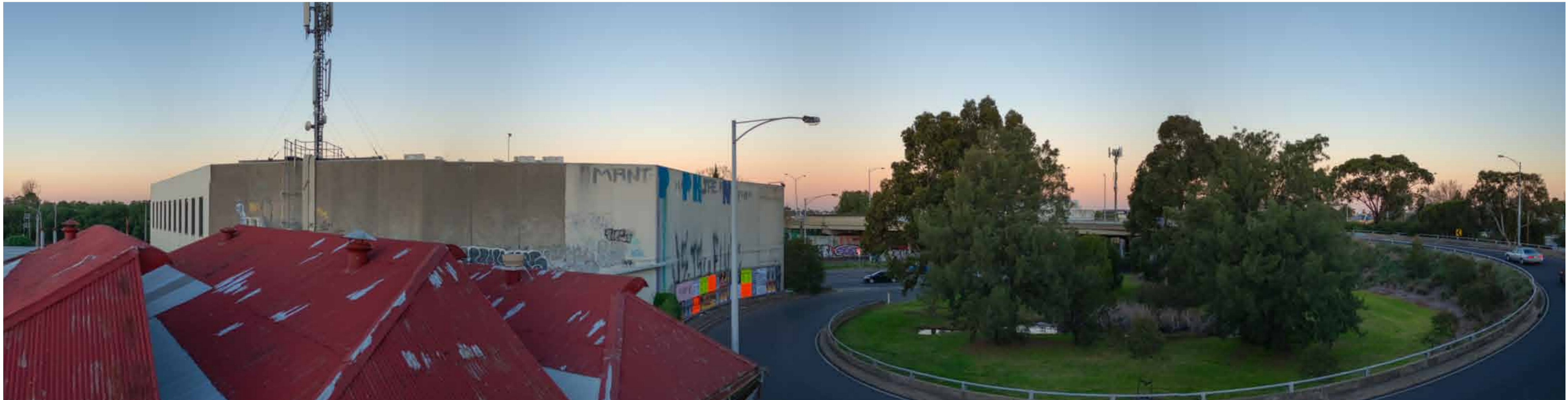
Level 2 South East View
