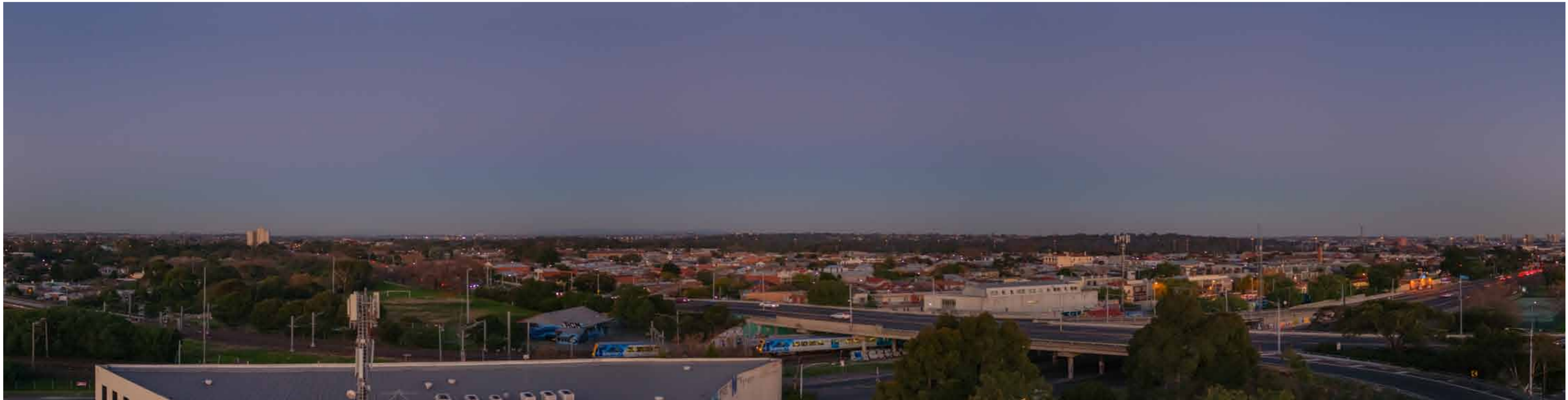
Level 8 South East View
