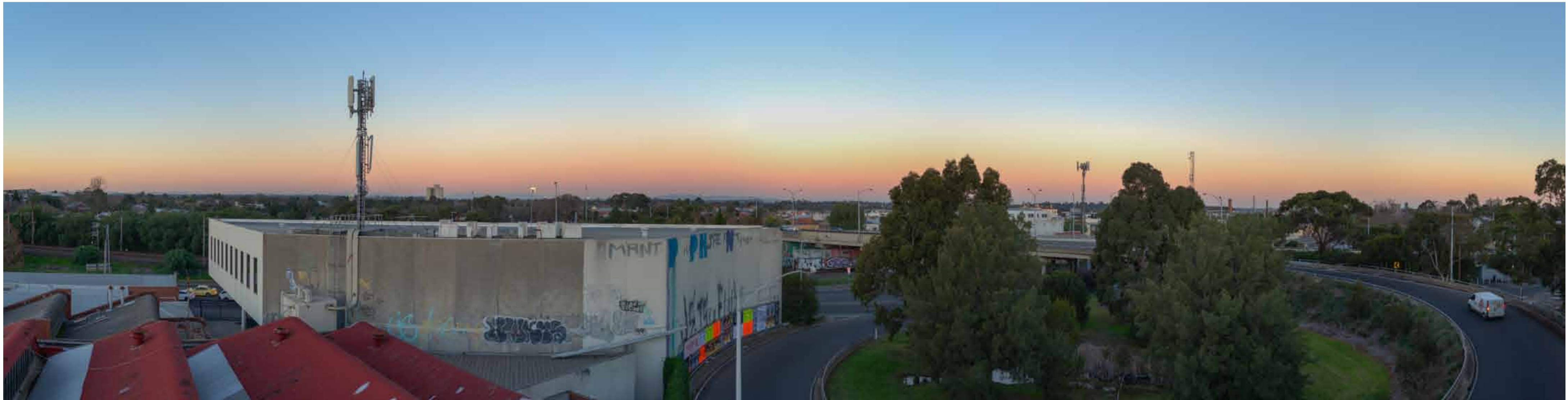
Level 4 South East View
