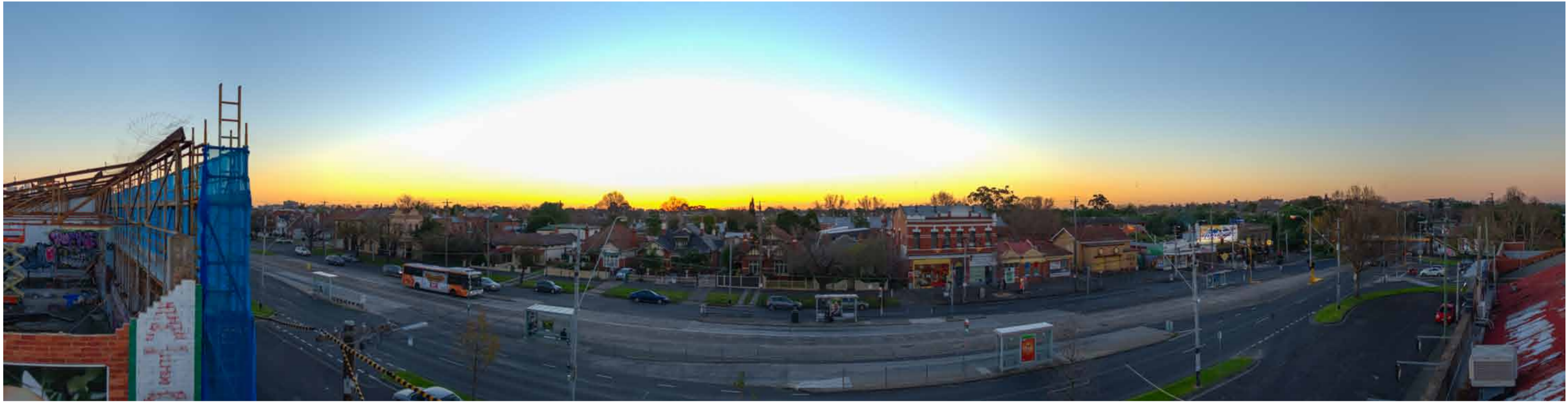
Level 3 South West View
