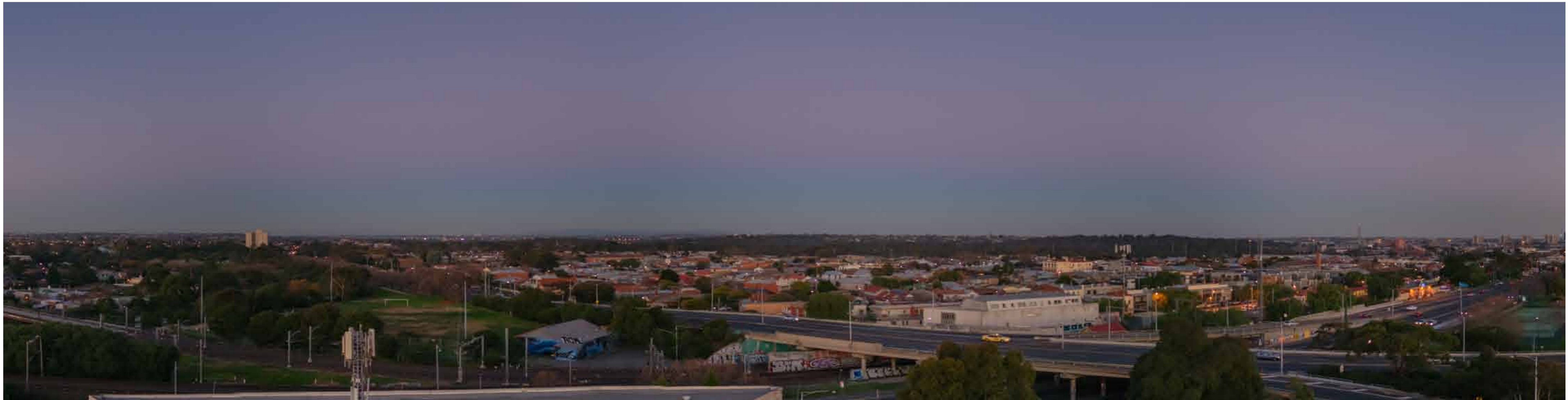
Level 9 South East View
